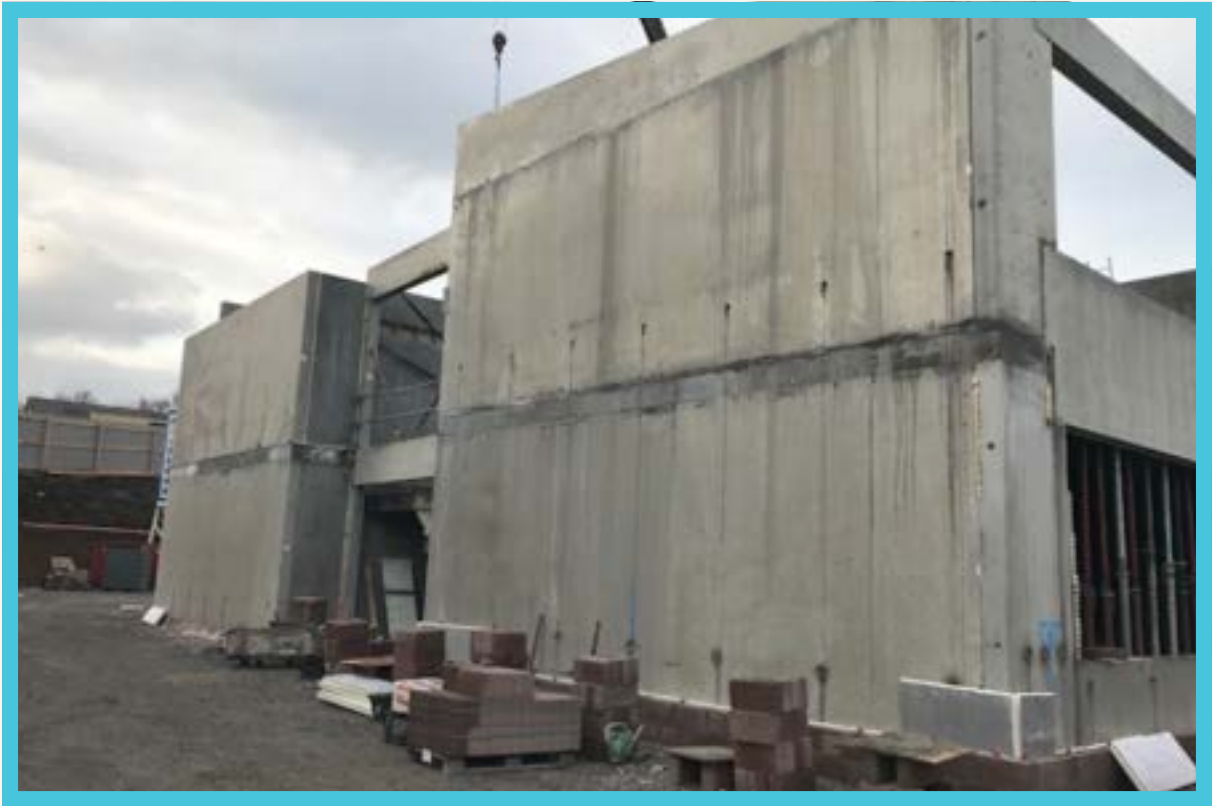
Figure 4: 2-D precast concrete walls being assembled.
