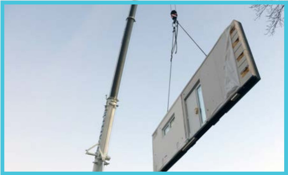
Figure 3: 2-D panel being hoisted onsite.
