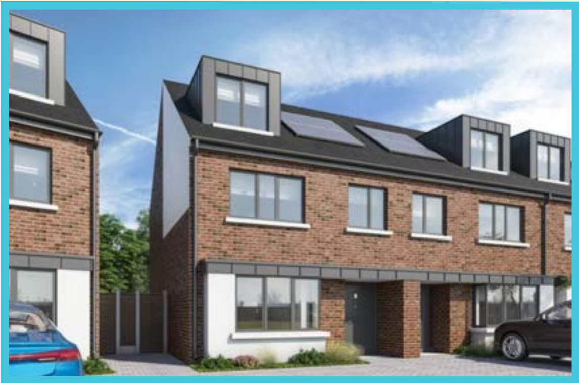
Figure 7: Timber frame building completed.
