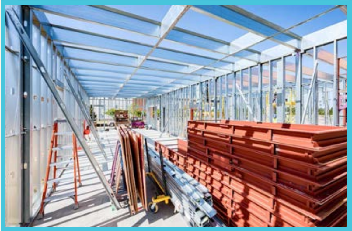
Figure 8: Light gauge steel framed building.
