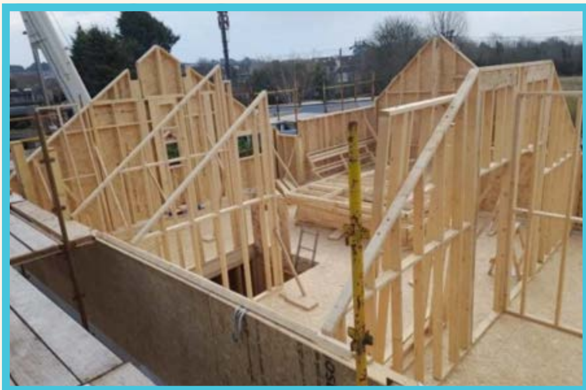
Figure 6: Timber frame building being erected.
