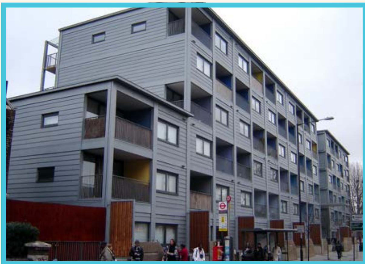
Figure 2: Modules stacked on a completed building.
