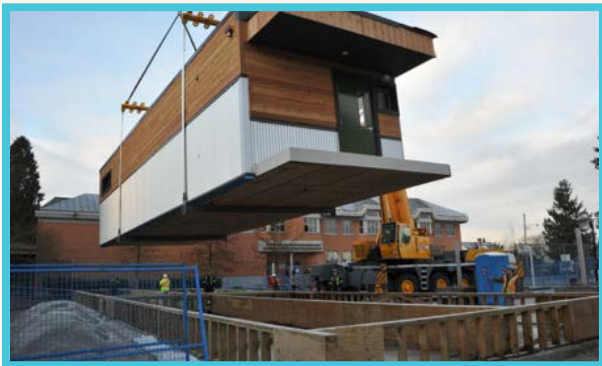
Figure 1: Module being hoisted onsite.
