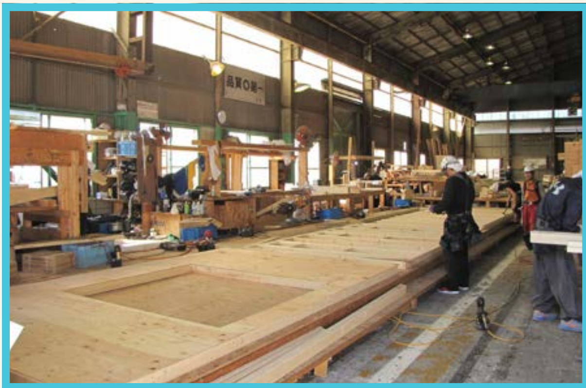
Figure 5: 2-D panel being built in a factory.
